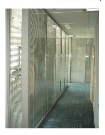
Partition system 570 - wall thickness 70 mm.
